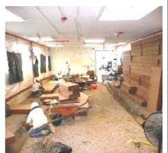
Park Range Construction was awarded the contract to **remove existing slab** on grade and install micropiles for a new concrete structural floor.
