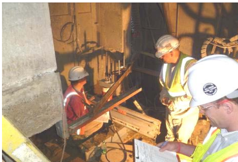
Engineers load-testing micropiles
