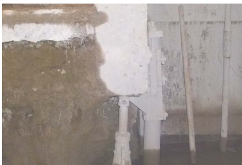
Micropile with underpinning bracket
