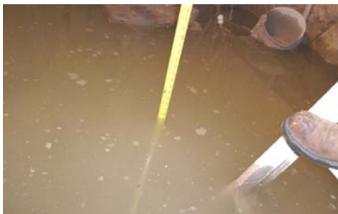
Dewatering required – 21” deep
